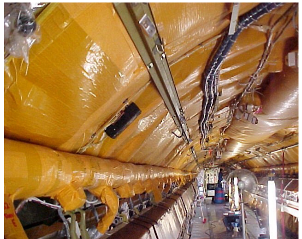
MPET insulation after installation of 3M™ Nextel™ Flame Shield AL-1.
