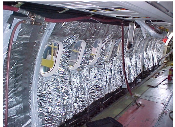
MPET Insulation before installation of 3M™ Nextel™ Flame Shield AL-1.
